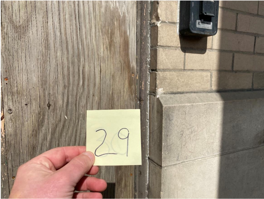
HA #29 – White Masonry Door Sealant
