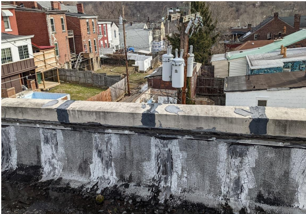
HA #15 – “End Cap Mastic” Mastic on top of Parapet Stone
