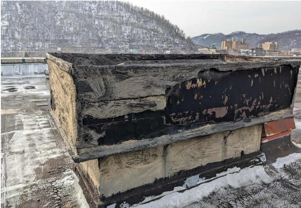
HA #16 – Mastic on Metal Duct, HA #17 – Pitch Pocket Mastic, HA #18 – Curb Flashing
