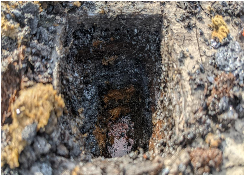
HA #11 – Rubber EPDM w/ Mastic, HA #12 – Built Up Roofing, HA #13 – Insulation Board
